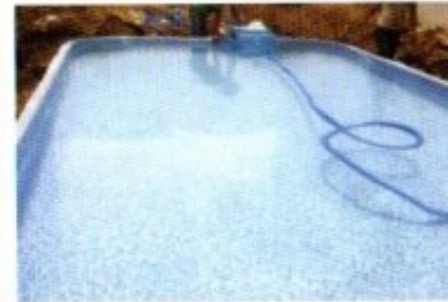
Prefab Pool at GHANDI NAGAR GUJARAT
