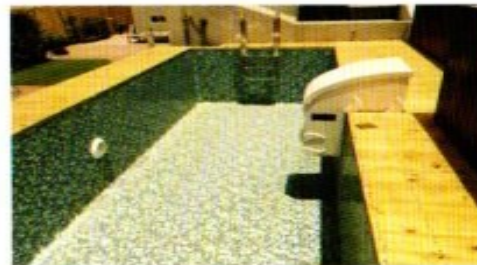
3. SUPPORT ALL AROUND NEEDED 600 mm extra space from swimming pool.
