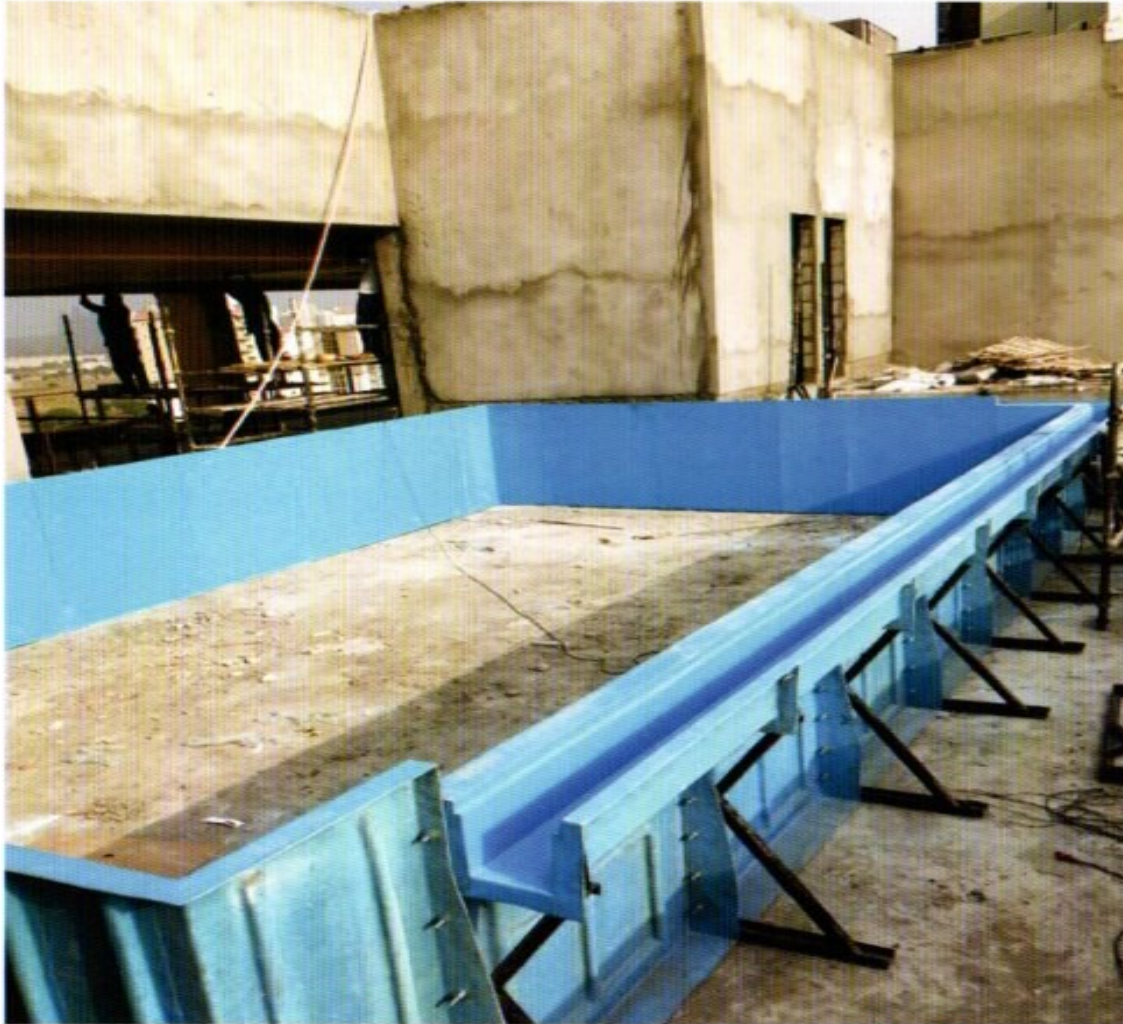
1. Step : Panels erecting
