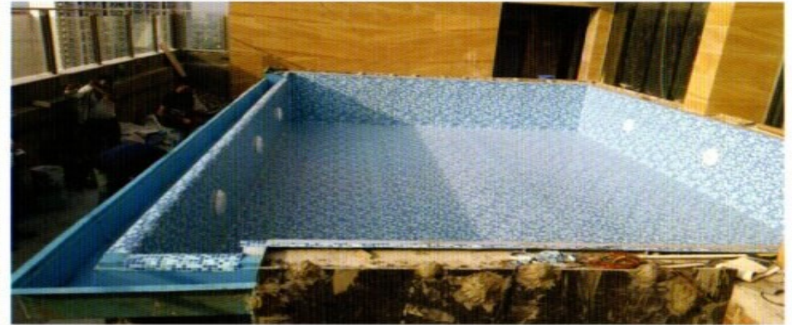
2. Pasting of Liner and Under water lights along with other fixtures.
